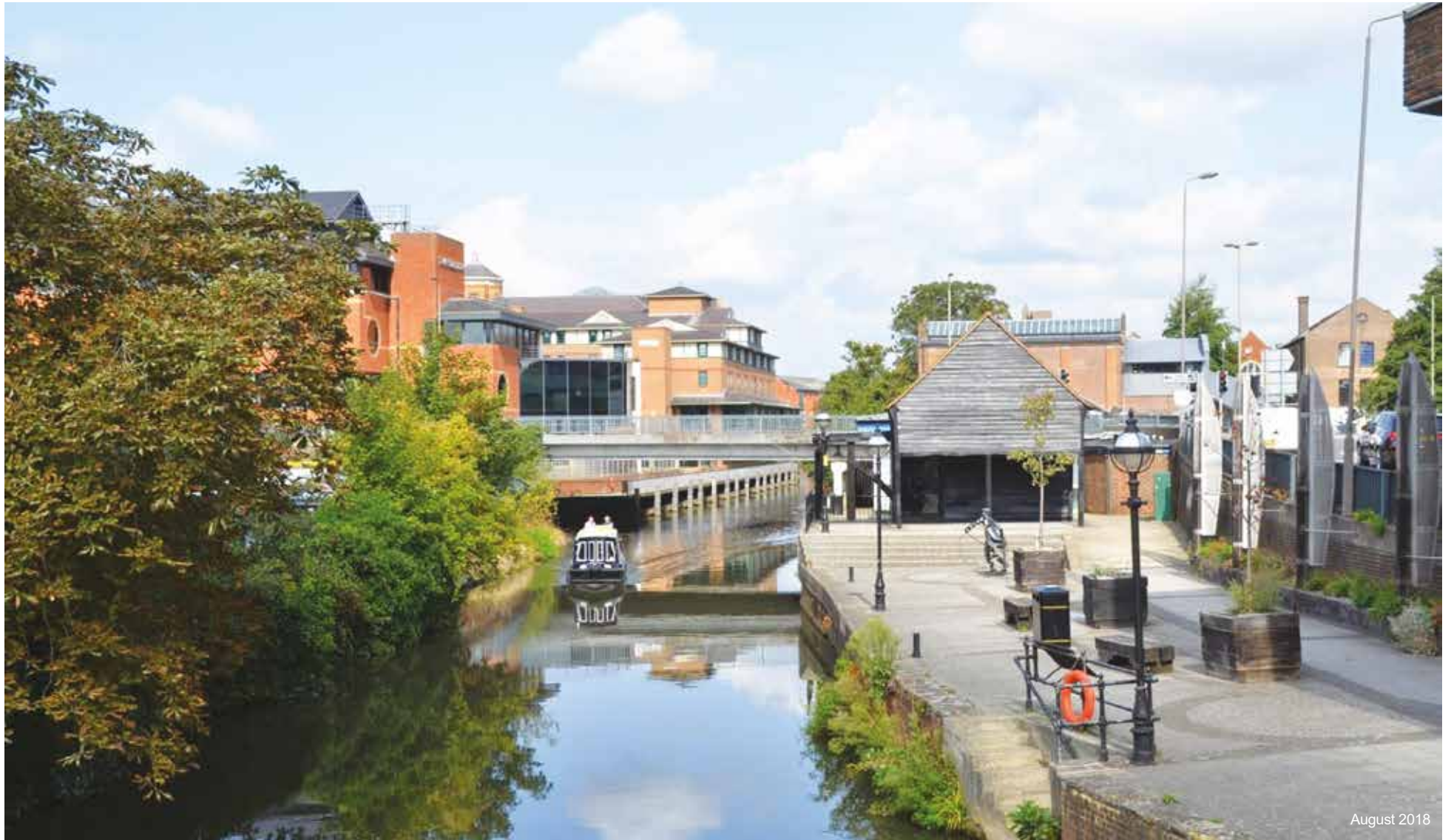
Fig. 5.13.11 Zoom view of the Treadwheel Crane on the bank of the River Wey
