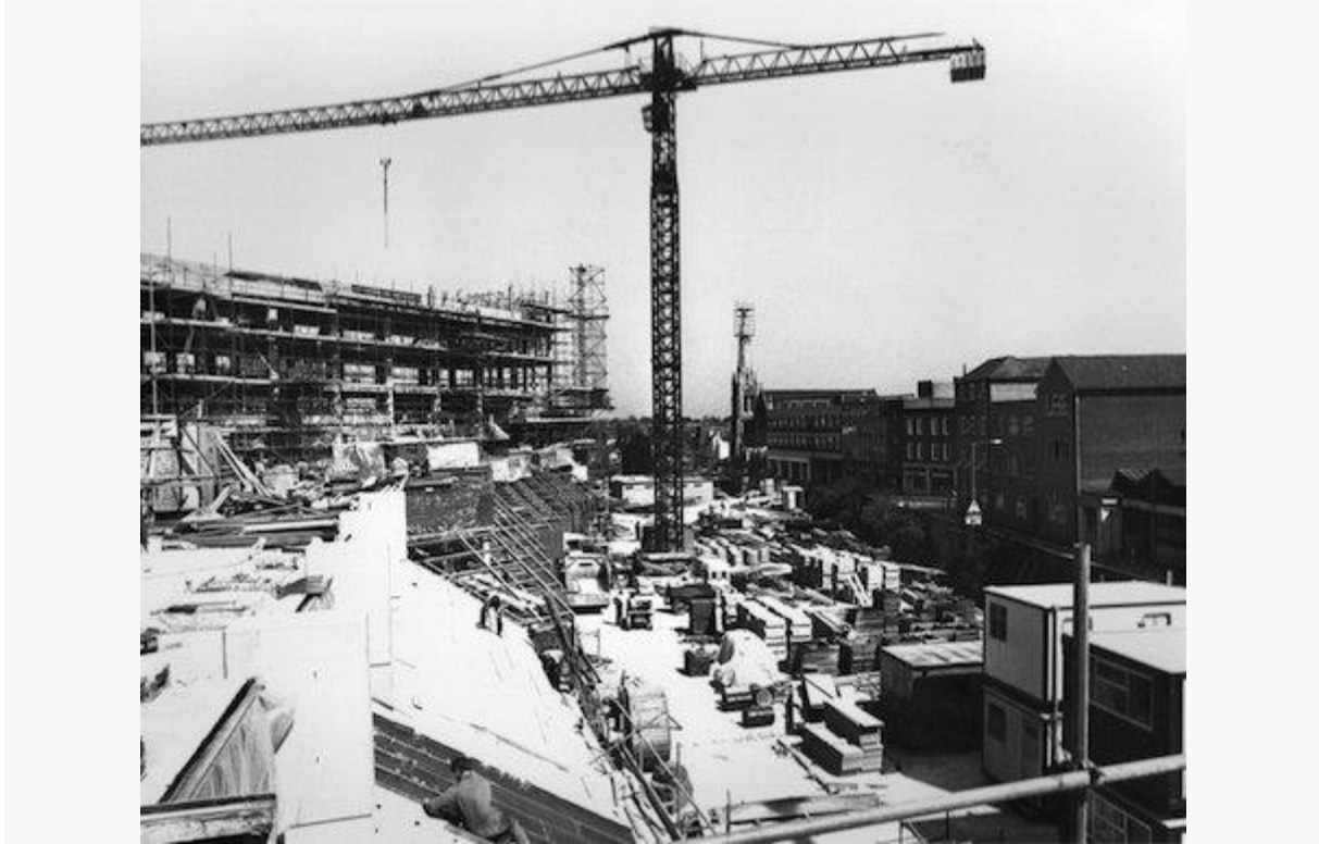
The Friary centre under construction.
