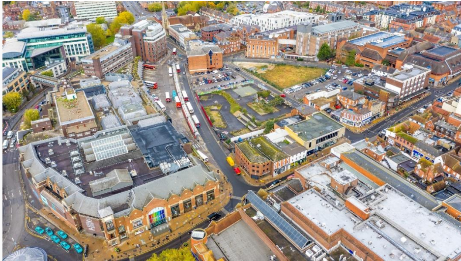
Aerial view of the North Street Regeneration site. Image – St Edwards
